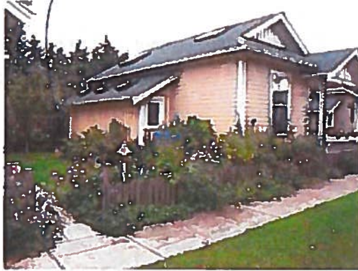
Closed side of the house – skylights bring light into the interior without peering at the neighbor
